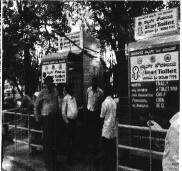
Smart E- Toilet Kasala shrestti Park
